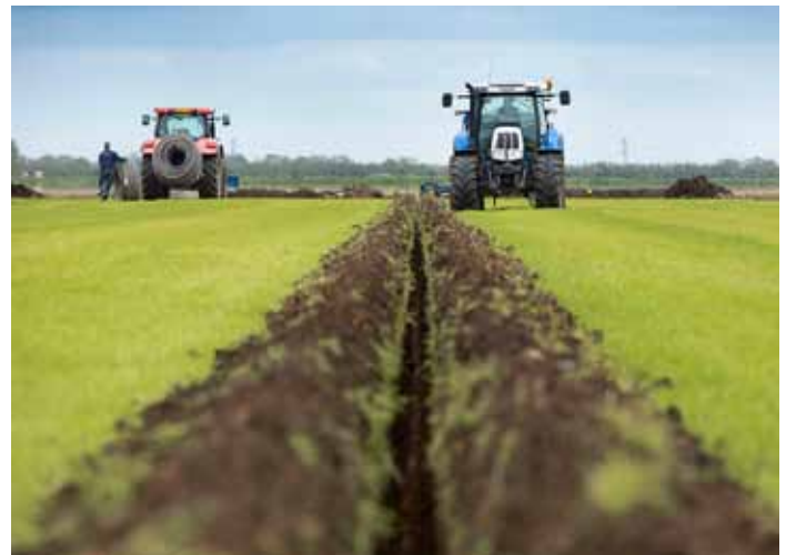
Figure 17 and 18. Construction of bio drain in The Netherlands (Source: Acacia Water, 2016)
