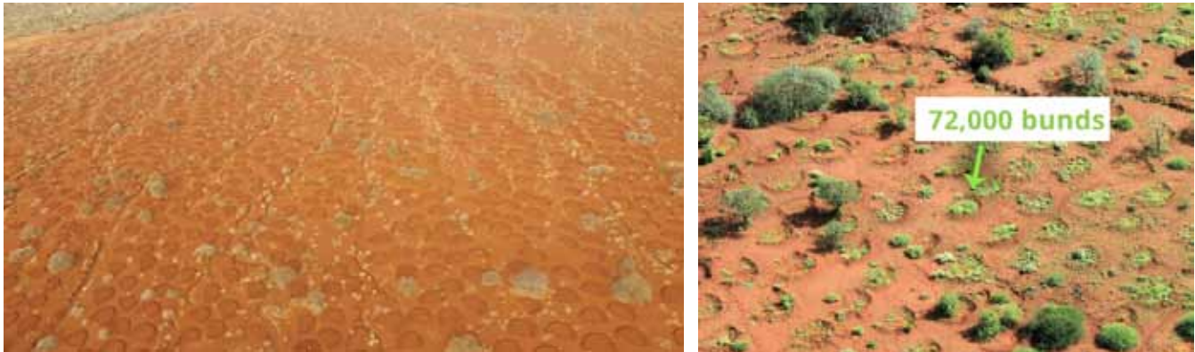
Figure 27. Micro-basins in Kuku, a) during construction and b) after one year (Source: Justdigg, 2017)
