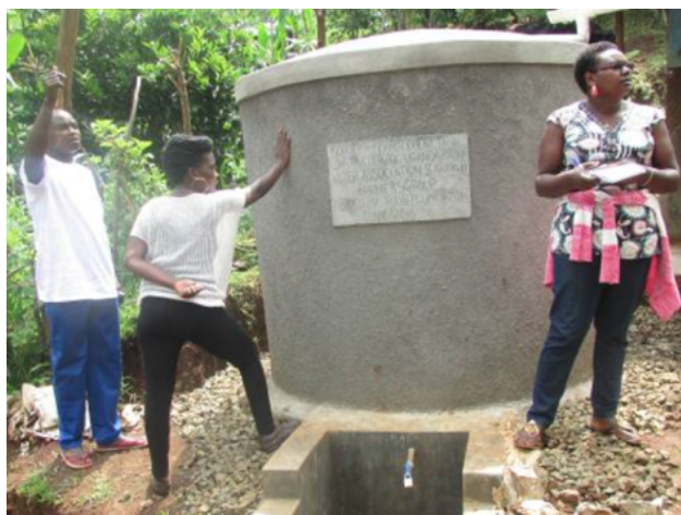
Figure 10. A ferro-cement tank (Source: URWA, 2017)
