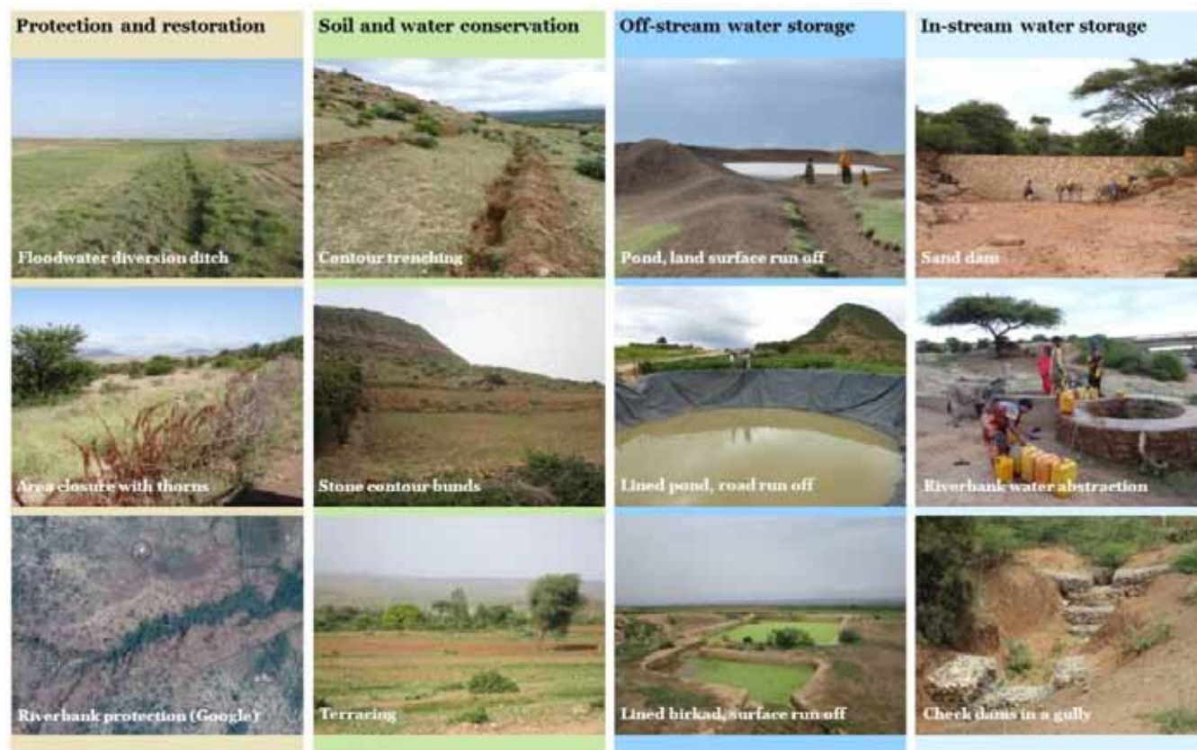
Figure 1. Variety of 3R measures that can buffer water highs and lows (Source: Acacia Water, 2017)
