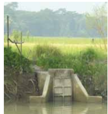
Figure 21. Gated culvert
