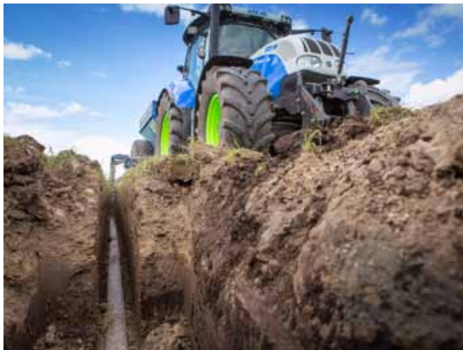
Figure 17 and 18. Construction of bio drain in The Netherlands (Source: Acacia Water, 2016)
