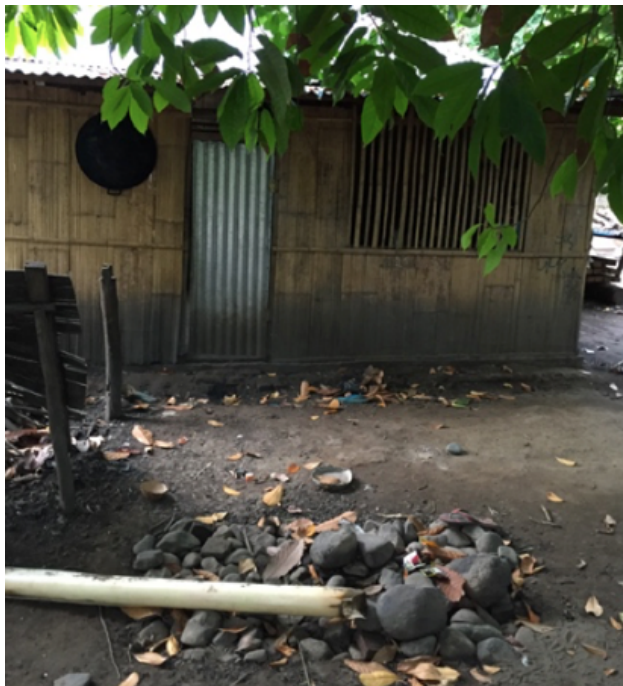
Figure 32. Infiltration pit filled with stones that allows floodwater to drain to more permeable layers (Source: RAIN)
